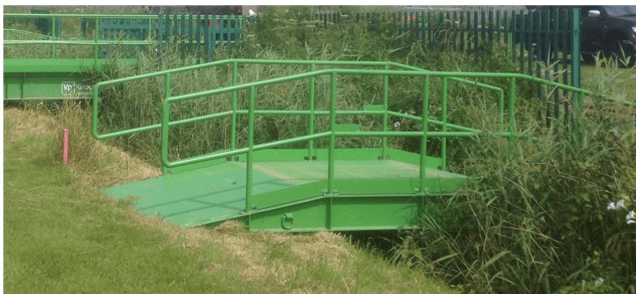
Figure 1.3 Indicative Temporary Ditch Crossing Bridge
